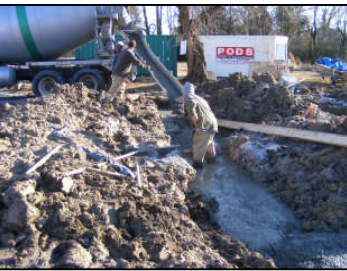
Steel Reinforced Concrete
