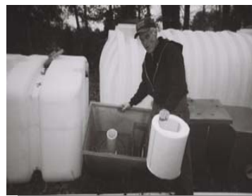
Prior to their installation, Southeast RCAP Technical Assistance Provider Douglas W. Phillips, Jr., P.E. shows some components of the potable rainwater system: the roof wash collection unit and filter and the storage tanks in the background.
